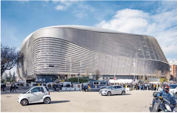
Refurbishment of the Santiago Bernabéu Stadium
