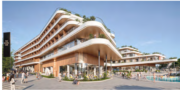
Hotel The Social Hub, en Cascais, Portugal
