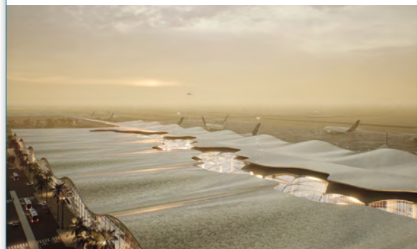
King Khalid Airport, Riyadh, Saudi Arabia
