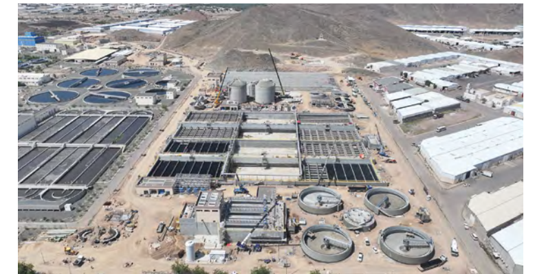
Medinah wastewater treatment plant, Saudi Arabia
