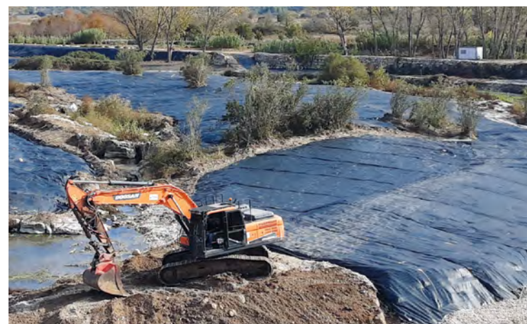
Restoration of riverbeds of the Jucar basin
