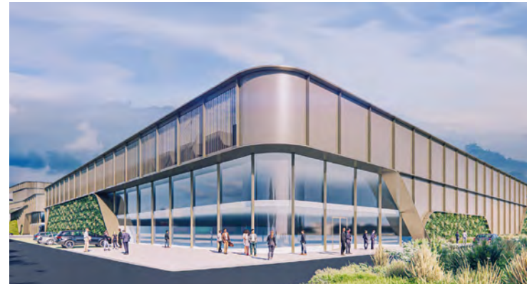
Goodman Data Centre in Amsterdam, The Netherlands
