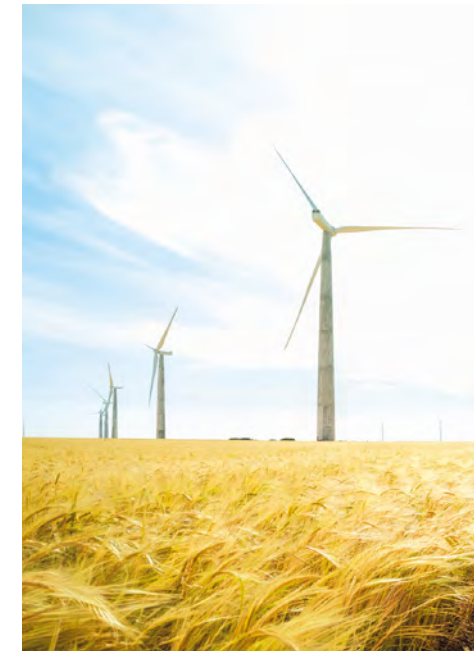
Existing GECAMA wind farm, Minglanilla, Cuenca
