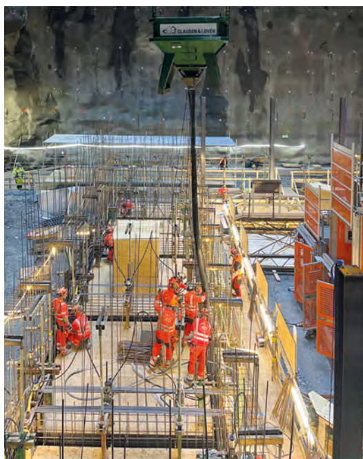
Stockholm Metro works. Blue Line
