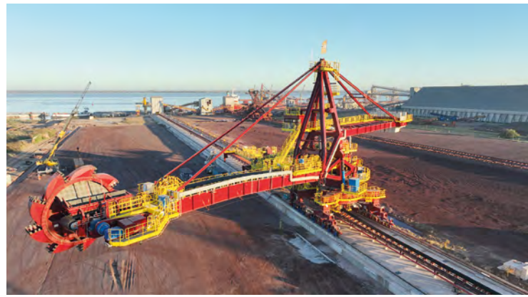
Bulk terminal at the Port of Nueva Palmira, Uruguay
