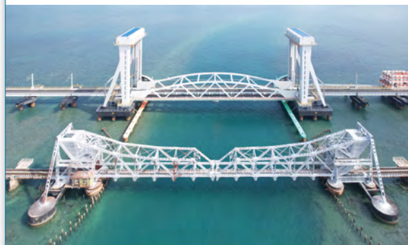
Pamban vertical lift railway bridge, India
