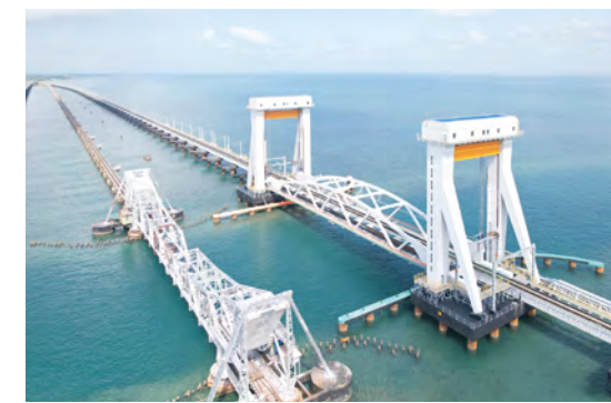
Pamban vertical lift railway bridge, India
