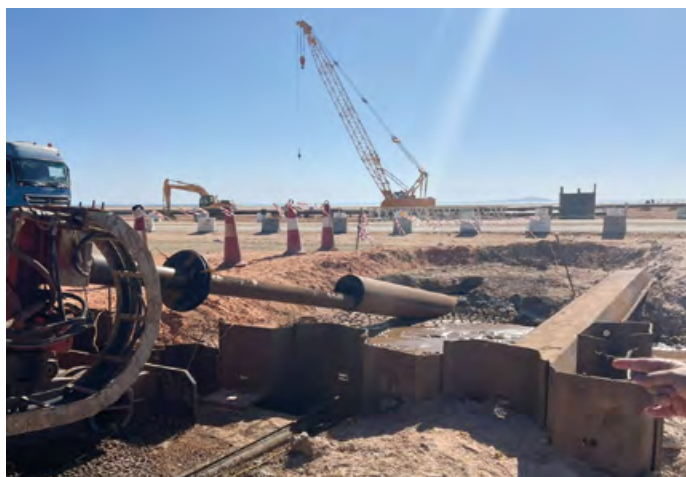
Horizontal drilling in NEOM to install submarine cable. Saudi Arabia
