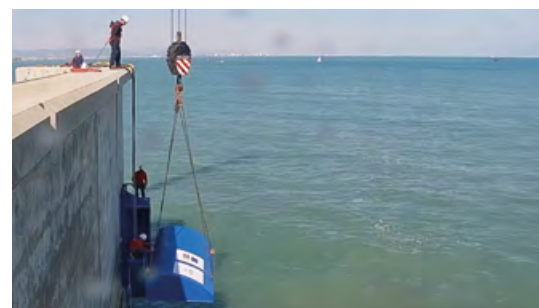
Installation of the wave energy device at the Port of Valencia
