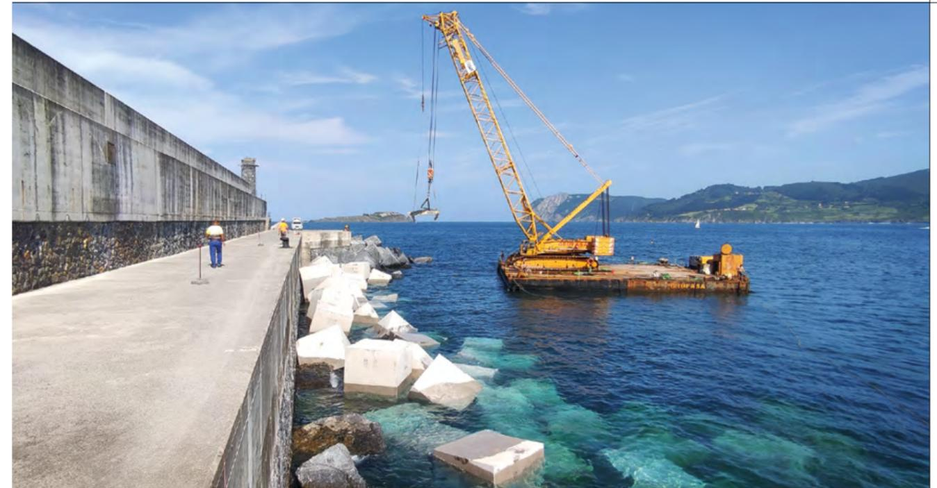
Construction supervision included breakwater reinforcement in the port of Bermeo, where siderurgical aggregate was incorporated during concrete manufacture to produce high-density concrete blocks. The use of this type of concrete achieves a positive environmental impact by reducing calcareous aggregate and creating value from electric furnace steel plant waste.
