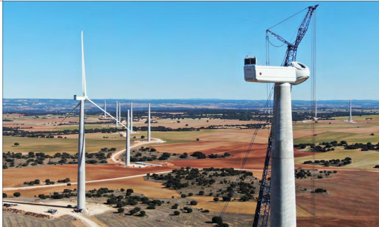
46 | Occupying an area of approximately 8,000 hectares, the farm is located in the province of Cuenca, between the municipalities of Honrubia, Atalaya del Cañavate, Cañada Juncosa and Tebar. The farm is made up of 69 wind turbines each with a power of 4.8 MW. The concrete tower has a hub height of 120 m, and the 149 m diameter rotor brings the total height of the wind turbine to almost 200 m.
