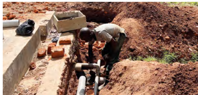
Drinking water supply works at UNILAC
