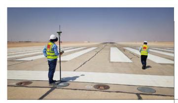
The aim of the project is to refurbish and upgrade the pavements on the two existing runways, 15R-33L and 15L-33R, on taxiway A, parallel to the secondary runway, and on 30 entry and exit taxiways (A, G and H at the ends of the runway, and entry and exit taxiways G1 to G7, A1 to A7 and H1 toH4). These actions will maintain safety levels and optimise the operational efficiency of the airport.
