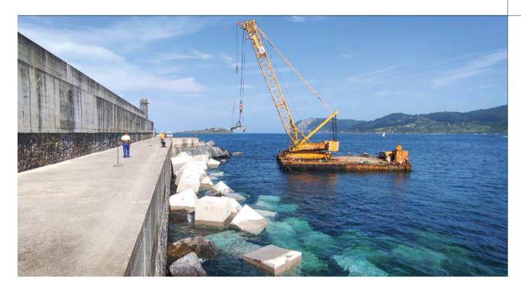
Construction supervision included breakwater reinforcement in the port of Bermeo, where siderurgical aggregate was incorporated during concrete manufacture to produce high-density concrete blocks. The use of this type of concrete achieves a positive environmental impact by reducing calcareous aggregate and creating value from electric furnace steel plant waste.
