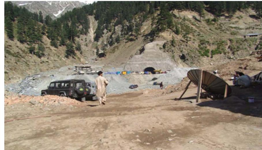
The tunnel is excavated following the NATM (New Austria Tunnelling Method) consisting in a continuous geotechnical evaluation and implementing the corresponding supports: shotcrete and wire mesh, lattice girders, bolting and reinforced concrete lining.
